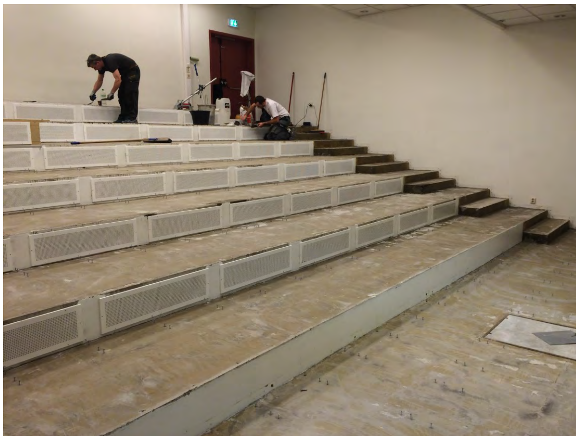
Store auditorium i Kallerudbygg II (Statped) under renovering.
