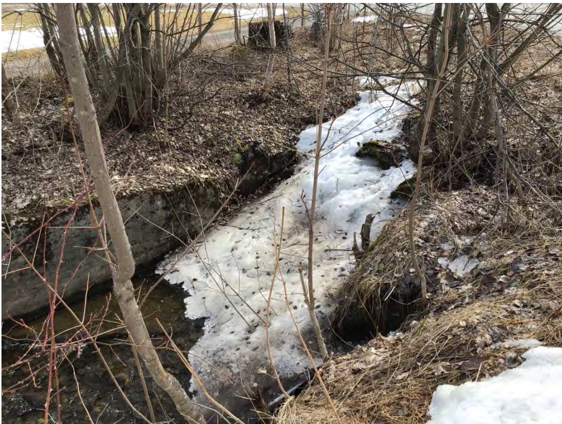
Figur 23 Kulvert 4 (1,0 meter og 1,0 meter)
